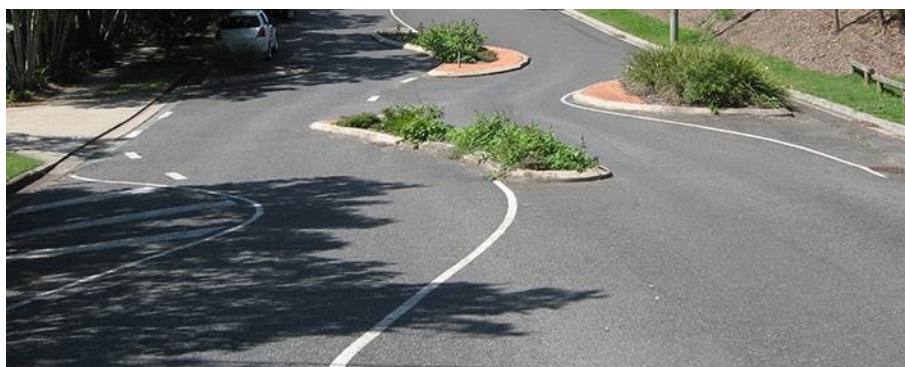
Figure 3.10. Speed limitation by chicanes.
