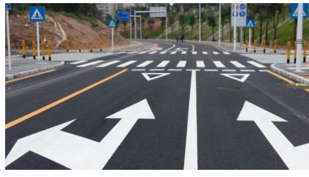
Figure 3.6. Road signs drawn on the road pavement.
