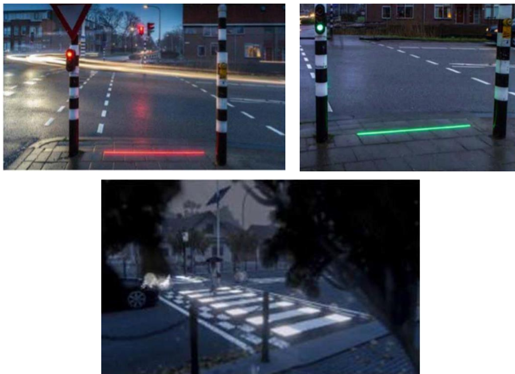
Figure 3.20. Smart pedestrian crossing.
