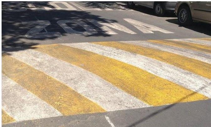
Figure 3.7. Elevated pavement speed limiter.
